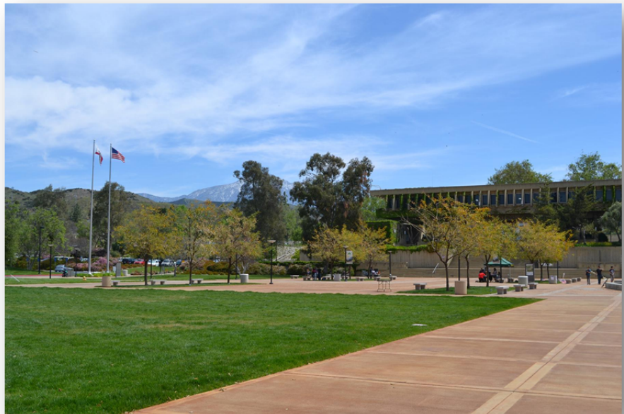
Crafton Hills College Laboratory/Administration Building
