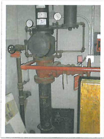
Fig 24 - Aeronautics Lab - 6" fire riser
