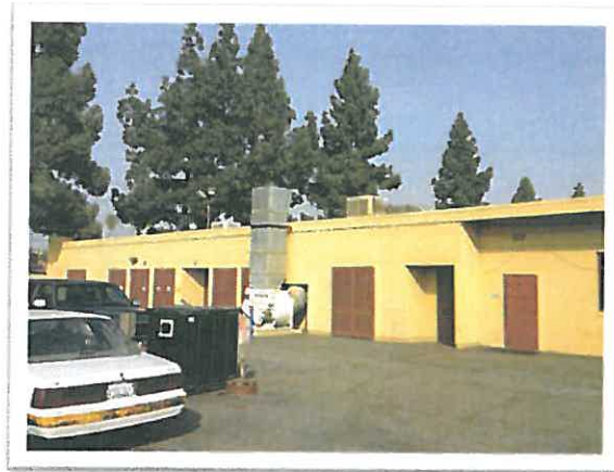
Figure M-5 - Exterior View of Welding 121 and Welding 12
