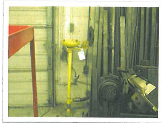
Fig 21 - Machine Shop – obstruction around emergency equipment and near electrical receptacle.
