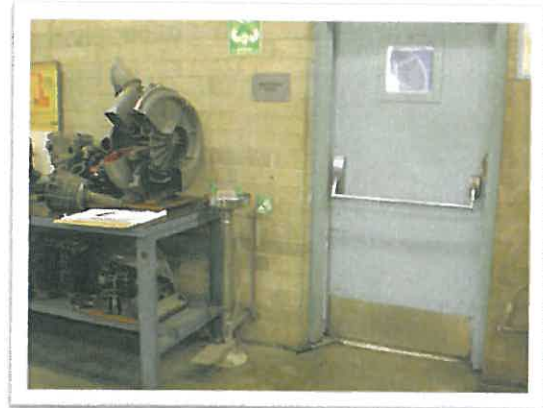
Fig 12 - Galvanized pipe supply with no backflow or check valve.
