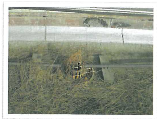
Fig 17 - Condensate drains terminating at a roof drain.
