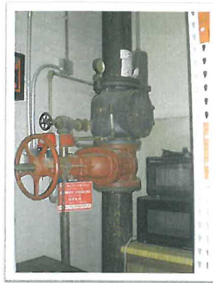
Fig 25 - Aeronautics Lab – 8" fire riser
