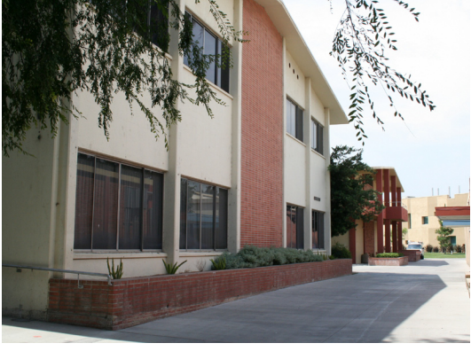
Chemistry Building - To be Demolished
