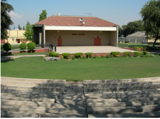
Planetarium - Recommended for Demolition.
