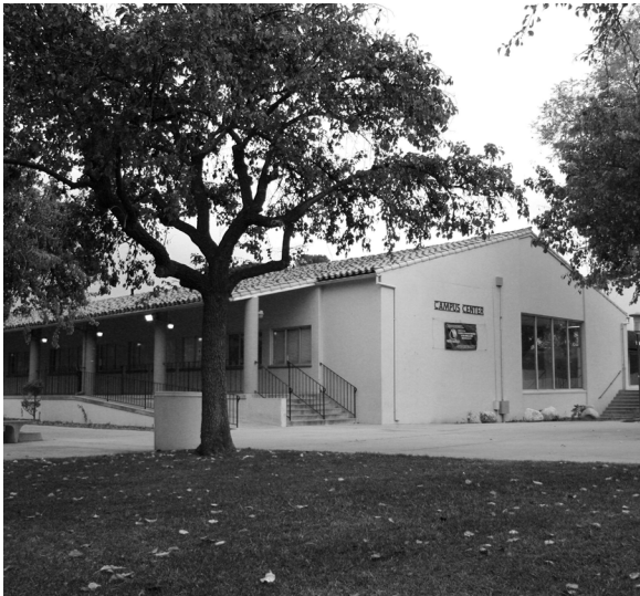
Campus Center - Demolished
