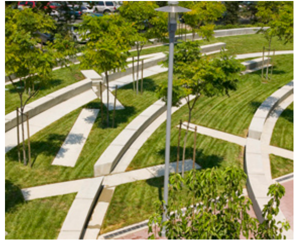
Retaining walls that double as benches along a sloped site University of California at San Francisco / San Francisco, CA
