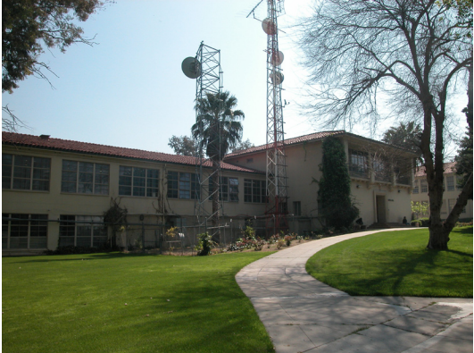
North Hall Building - To be Demolished
