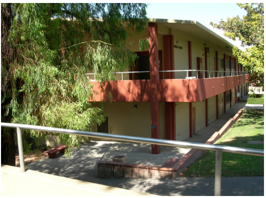
Physical Science Building - To be Demolished
