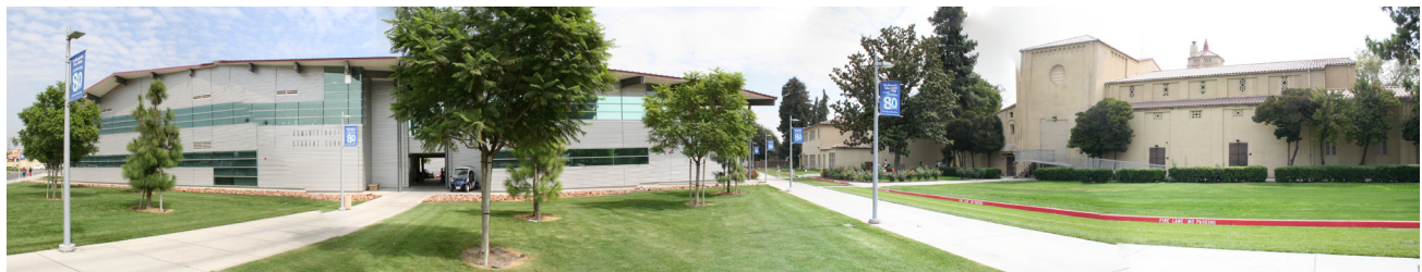
Bridging the gap - the Administration/ Student Services building and the Auditorium
