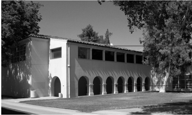
North Hall - To be demolished
